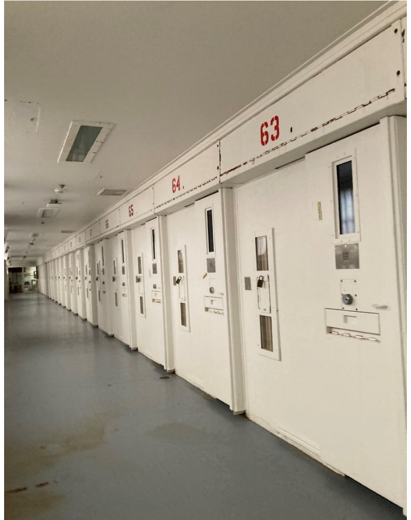
Former solitary confinement cells at Washington State Reformatory at Monroe Correctional Complex
