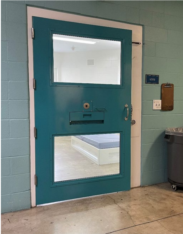
Updated cell door in Close Observation Area at Monroe Correctional Complex (2024)
