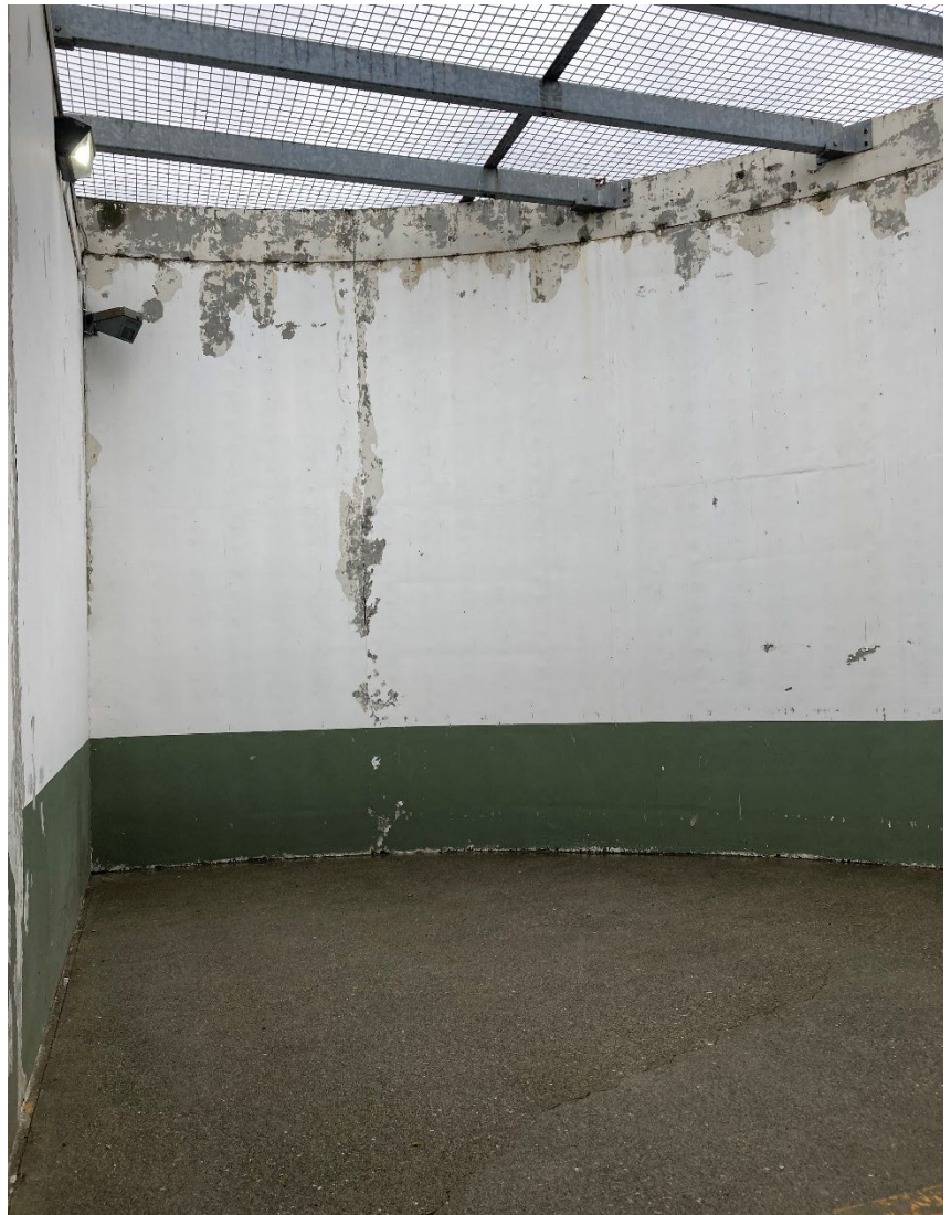
Image 20: Outside yard for solitary confinement at the Residential Treatment Unit (RTU) at Monroe Correctional Complex Sky River Treatment Center (MCC-SRTC).
